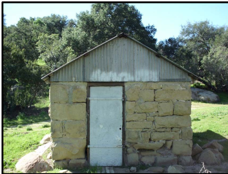
Figure 1 Old Powder House (East Elevation) Facing West Source: URS Corporation, 2013.
