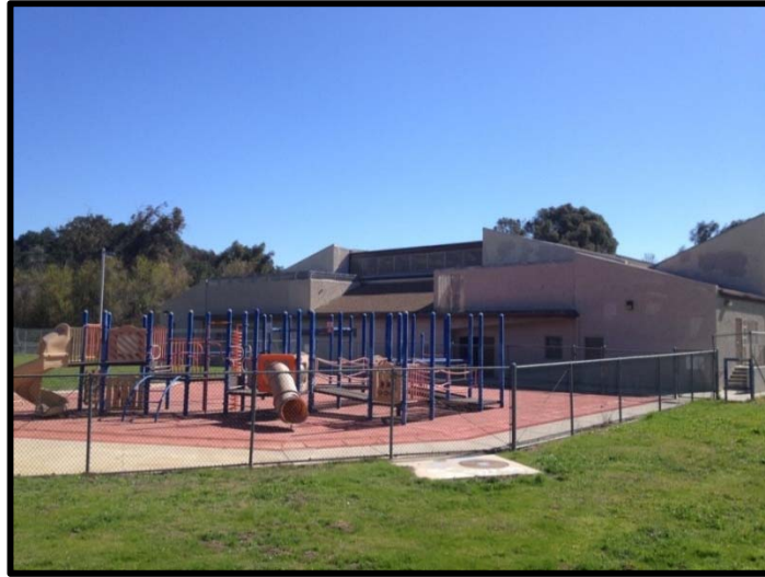
Figure 3 View of Existing North Playground Facing Southeast Source: URS Corporation, 2013.
