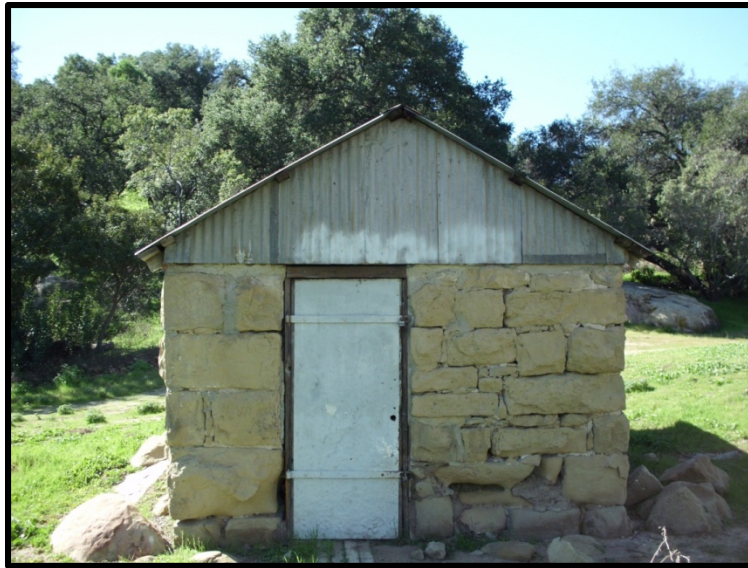
Figure V-A Old Powder House (East Elevation) Facing West Source: URS Corporation, 2013.
