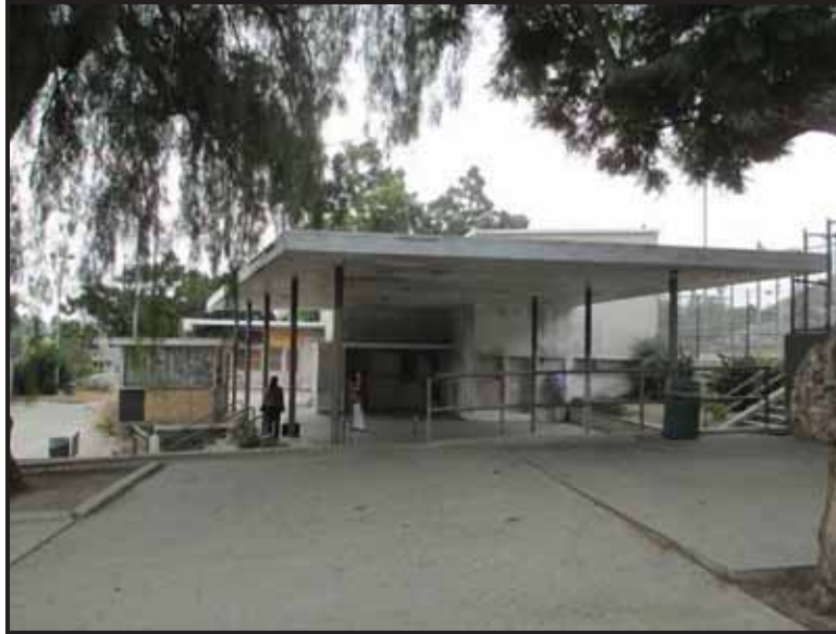
Figure 5. Recreation Clubhouse, view facing south.
