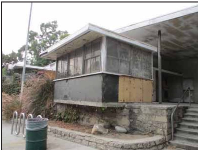
Figure 6. Concession Stand, view facing southwest.
