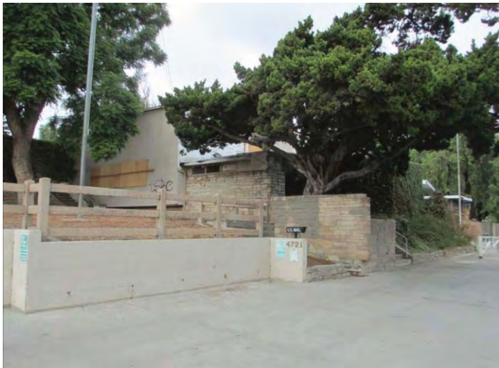
South elevation, view facing northwest.
