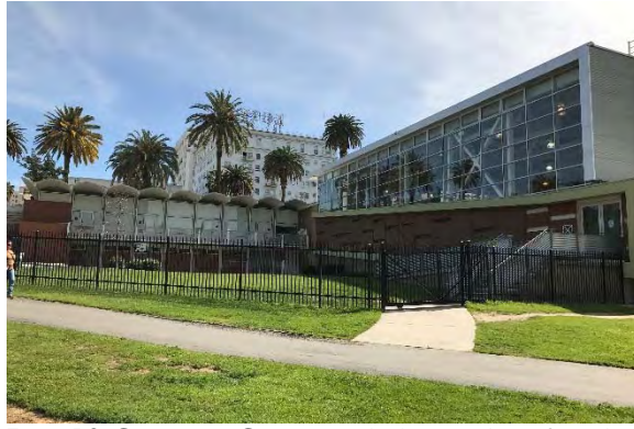
Figure B8: Community Center, view looking southeast from the Project Site, March 2017 (Historic Resources Group)
