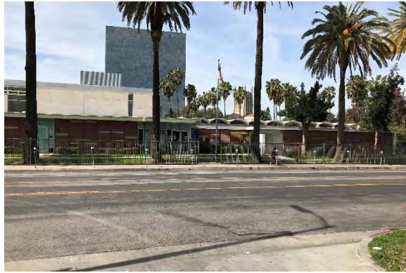
Figure B10: Community Center, east (primary) façade, March 2017 (Historic Resources Group)
