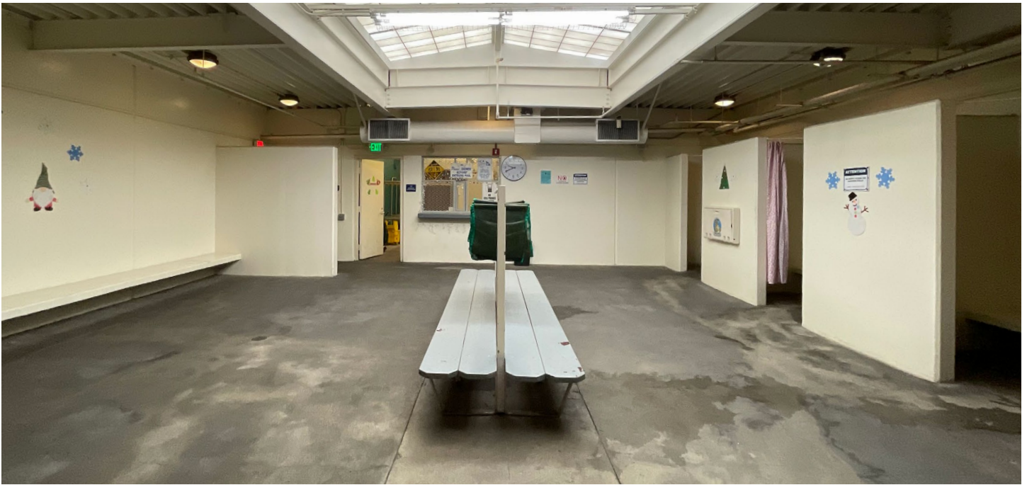
Current Conditions Women's Locker Room, Echo Park Indoor Pool
