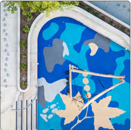
High Density Rubber Surfacing 0.5-1.5mm particle size Upcycled content Custom graphic
