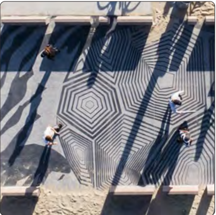
Etched C.I.P. Concrete Cast in place with color sealant Sandblast etch graphic
