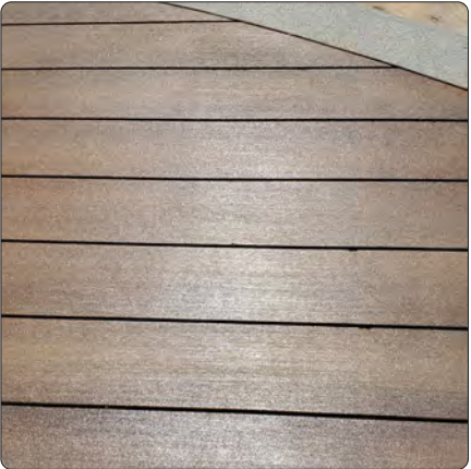
Faux Wood Decking Cast in place concrete with specialty wood finish 6" joint spacing, typ.
